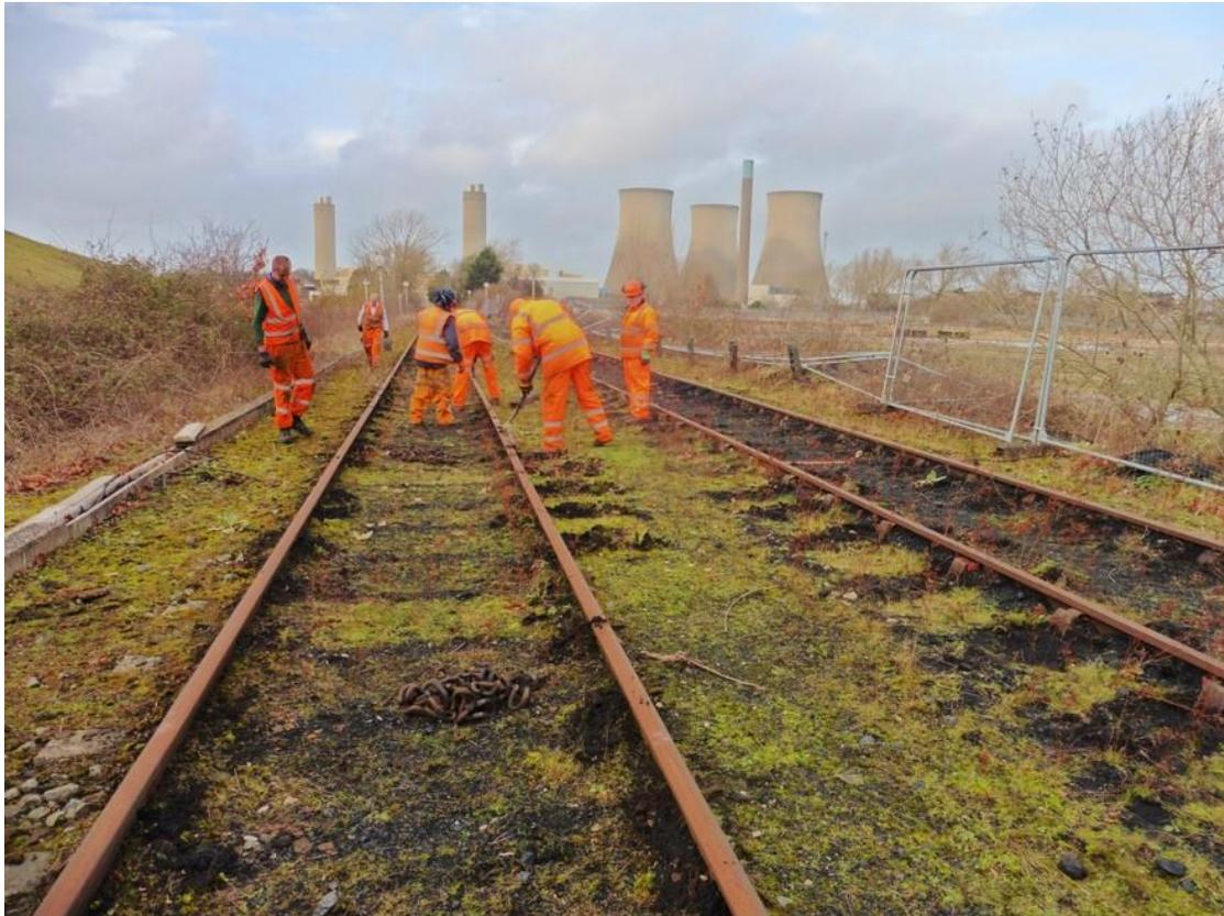
***Removing the e-clips from one of the former Didcot coal loop departure lines. The coal unloading bays were located around to the left in the far distance.***
